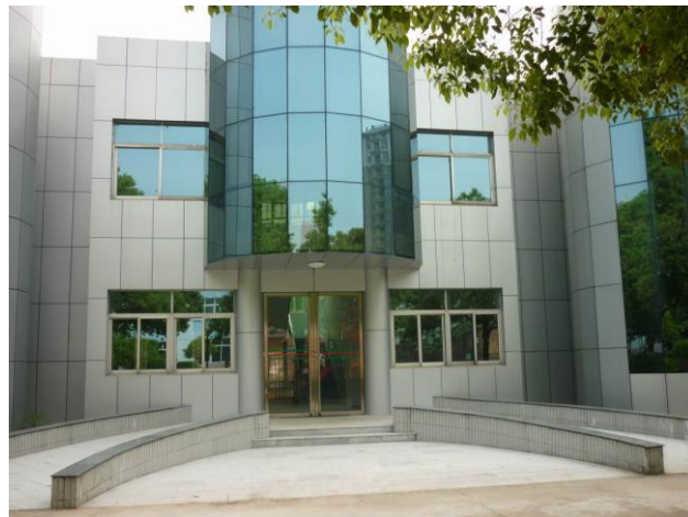
The soon to be completed rehabilitation center.
